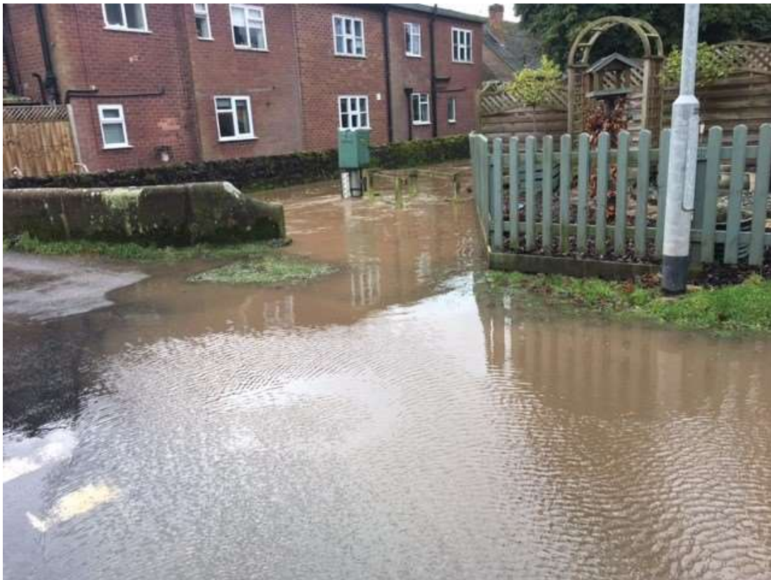
Flooding at Church Lane road bridge, Marchington
